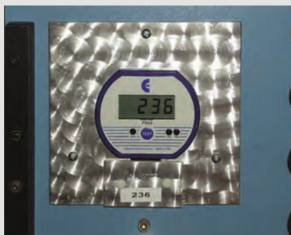
Pipe Pressure Testing System
