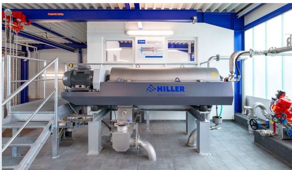
Hiller decanter in municipal wastewater treatment
