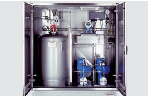
Flow proportional: precisely controlled odourant addition e. g. in the natural gas supply
