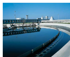
Wastewater process: biological water treatment.
