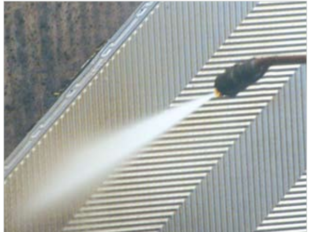
Thoroughly cleaned plates are essential for good PHE performance. Pressure washing of the stripped plates removes loosened material.
